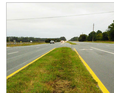
Looking northbound from the median at Bayford Road
