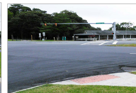
U.S. Route 13/Parksley Road intersection from southwest corner
