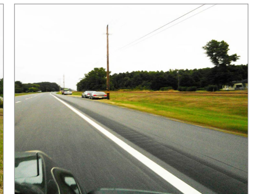
Vehicles parked on the eastern side of the northbound travel lane on U.S. Route 13
