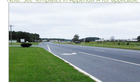
Northbound right turn lane onto Front Street from U.S. Route 13
