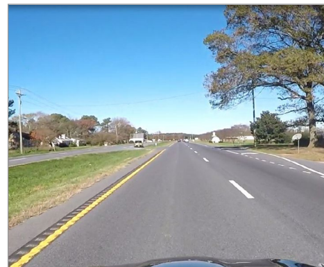
Vehicle traveling northbound on U.S. Route 13 approaching Thorton Road
