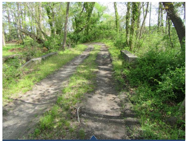
**Figure 4 -** A culvert that formerly carried the railroad remains and provides an option for the crossing of Old Plantation Creek
