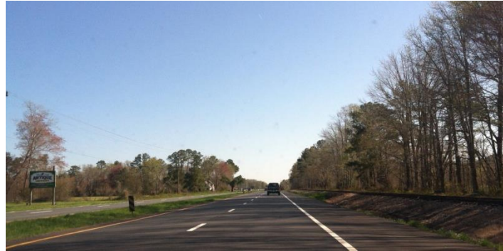
Figure 3, View of Paved, 6-foot Shoulder
