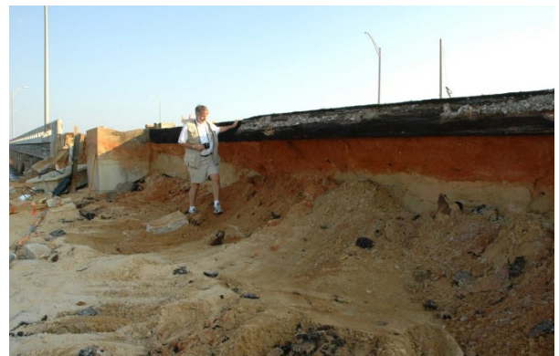
Figure 5 – Photograph of wave attack damage to embankment (from FHWA, 2014)
