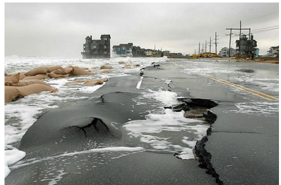
Figure 7 – Photograph of shoreline recession resulting in roadway damage (from FHWA, 2014)
