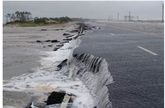
Figure 6 – Photograph of weir-flow damage mechanism as it occurs (from FHWA, 2014)
