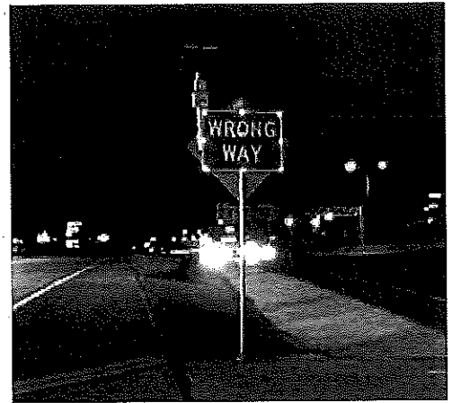
The LED-illuminated Wrong Way sign with radar is a standard wrong-way driver counter-measure on exit ramps in San Antonio.
