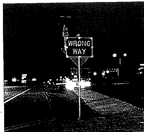
The LED-illuminated Wrong Way sign with radar is a standard wrong-way driver counter-measure on exit ramps in San Antonio.
