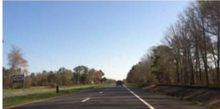
Figure 3, View of Paved, 6-foot Shoulder
