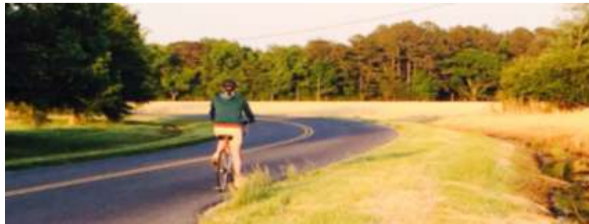
Figure 7, Eastern Shore Bicyclist on Road with Unpaved Shoulder and Nearby Ditch
