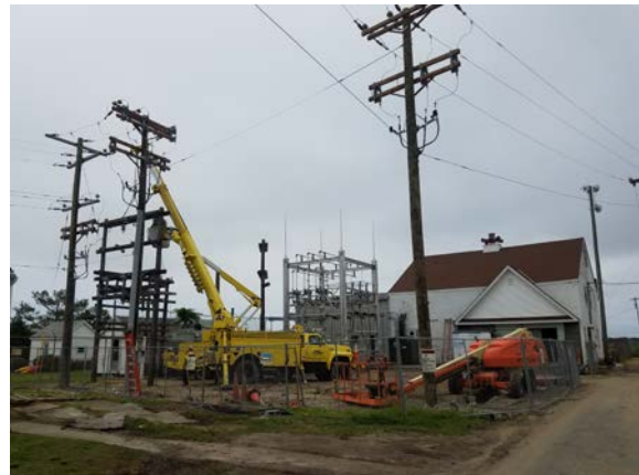
Figure 7: Electric substation. Photo by Shannon Alexander
