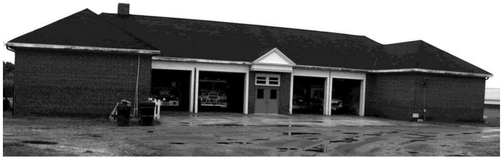
FIGURE 10.5 Saxis' firehouse and Town office located in a flood zone. Photo by Elaine Meil
