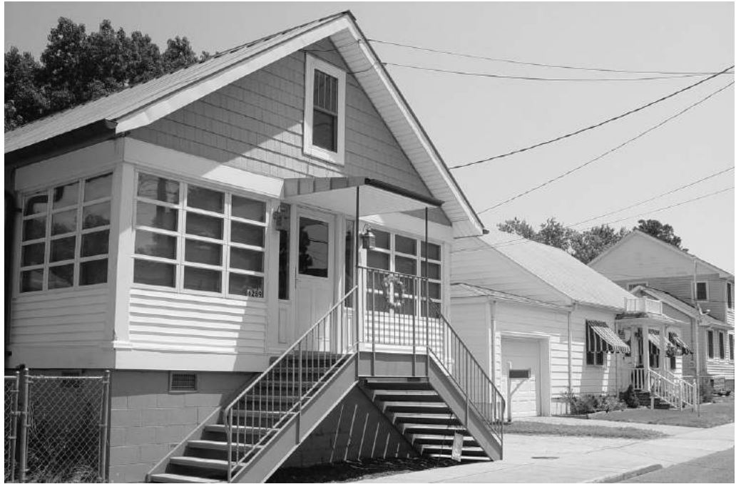
FIGURE 9.2 Chincoteague home elevation project.
