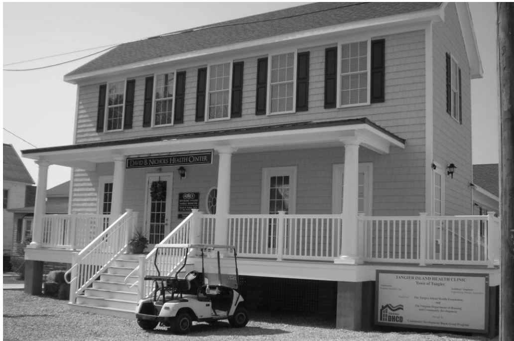
FIGURE 14.6 The Tangier Health Center was constructed in 2010 in a manner that minimizes impacts from flooding and high winds. Photo by Curt Smith
