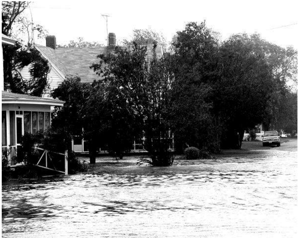
PICTURE 4.3 Homes in Wachapreague during Hurricane Isabel. These homes are located in an A zone with a Base Flood Elevation that includes a wave height component. Photo by John Aigner
