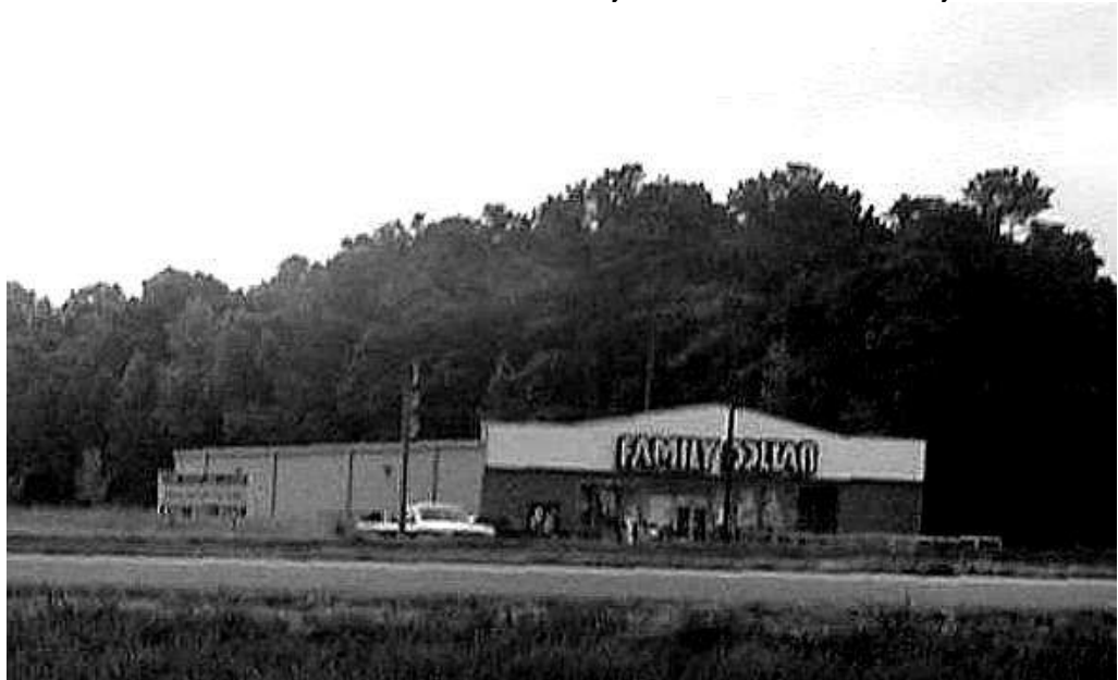
PICTURE 8.1 This building and its parking lot in the Town of Onley frequently is flooded by storm water. As can be seen from the truck in the picture this building was built in a substantial depression. Just visible in the photo is the platform for customers to access the store after a rain. The lot next door, also located in the depression, is for sale. Photo by Elaine Meil
