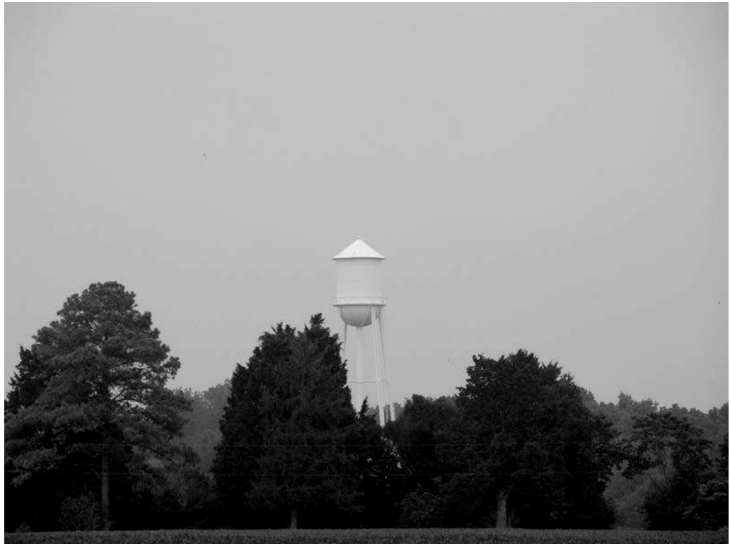
PICTURE 14.2 Water tower for the town of Eastville. Photo by Elaine Meil
