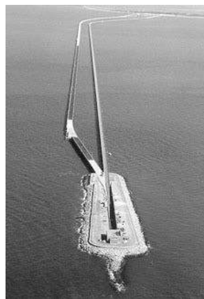
PICTURE 14.1 Chesapeake Bay Bridge Tunnel, the only southern road link to the Eastern Shore. Photo by Chesapeake Bay Bridge Tunnel Commission
