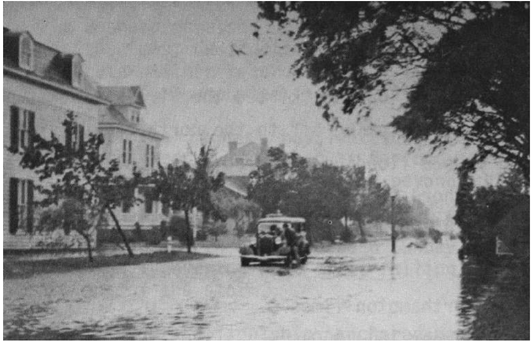
PICTURE 1.1 Flooding on Randolph Avenue, 3 ½ blocks from the Chesapeake Bay, in Cape Charles from one of the 1930s hurricanes. Photo printed in the Army Corp of Engineers Flood Plain Report for Cape Charles
