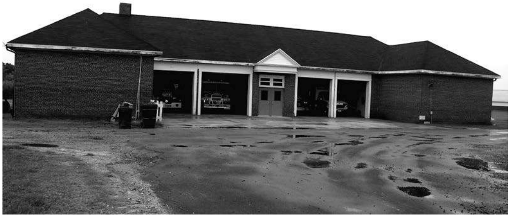
PICTURE 10.3 Saxis' firehouse and town office located in a flood zone. Photo by Elaine Meil
