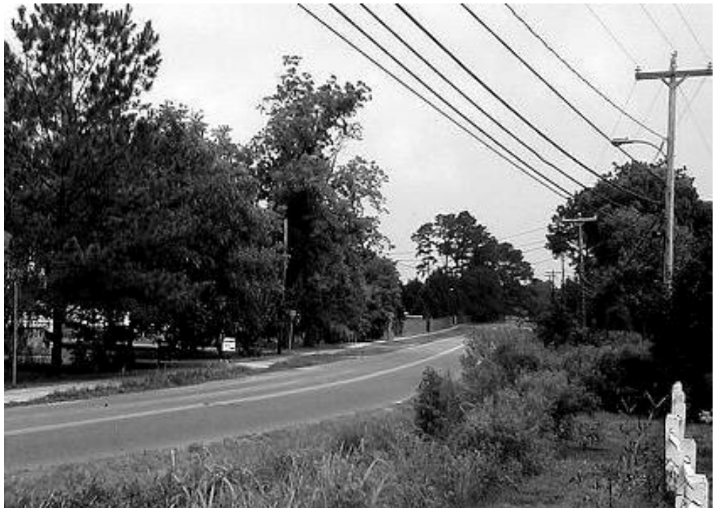
PICTURE 13.1 The fence in the distance is the Onancock Wastewater Treatment Plant. The home to the side of the picture has recently been elevated to the Base Flood Elevation. Photo by Elaine Meil
