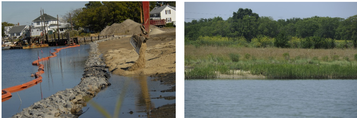
Figure 14: Living Shoreline in Oyster, Virginia. Left: October, 2009 - Construction. Right: July, 2012 - Fully Established. Photo Credit: Jay Diem, Eastern Shore News.
