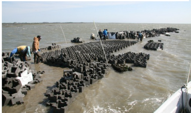
Figure 11: Oyster Reef under Construction Photo Credit: © Bowdoin Lusk/ The Nature Conservancy. Used with permission.
