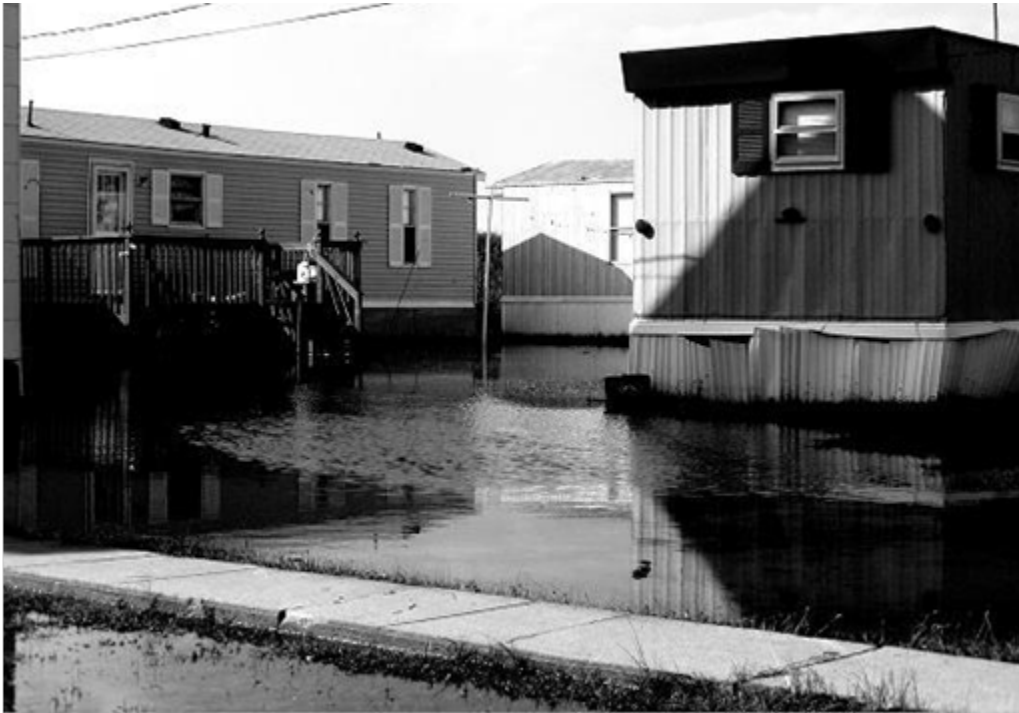
Figure 16: Flood water ponding around homes on Tangier after Hurricane Isabel in September 2003. Photo by Deborah Mills.
