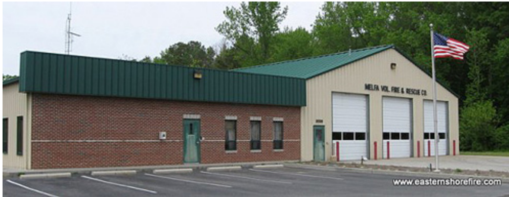
Figure 2 : Melfa Volunteer Fire and Rescue Company building on Hatton Avenue includes 3 bays, a community room, bunk rooms, restrooms, station watch room, laundry room, offices, & storage areas.
