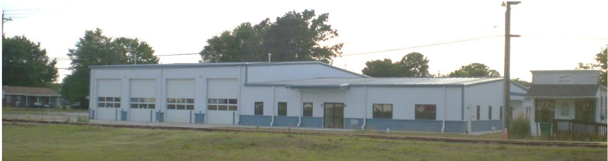
Figure 3: The new Fire and Rescue Department under construction in 2011. The railroad is a vital and historic component of the Town and can be seen in the foreground. Photo by Curt Smith
