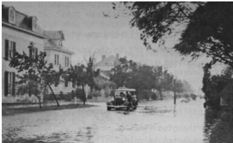
Figure 4: Flooding on Randolph Avenue, 3 ½ blocks from the Chesapeake Bay, in Cape Charles from one of the 1930s hurricanes. Photo Credit: U.S. Army Corps of Engineers Flood Plain Cape Charles Report
