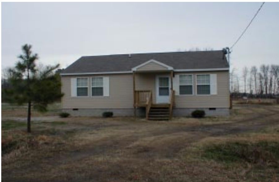
IPR Replacement House
