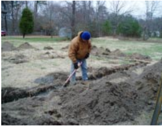
Contractor pouring Metompkin footings
