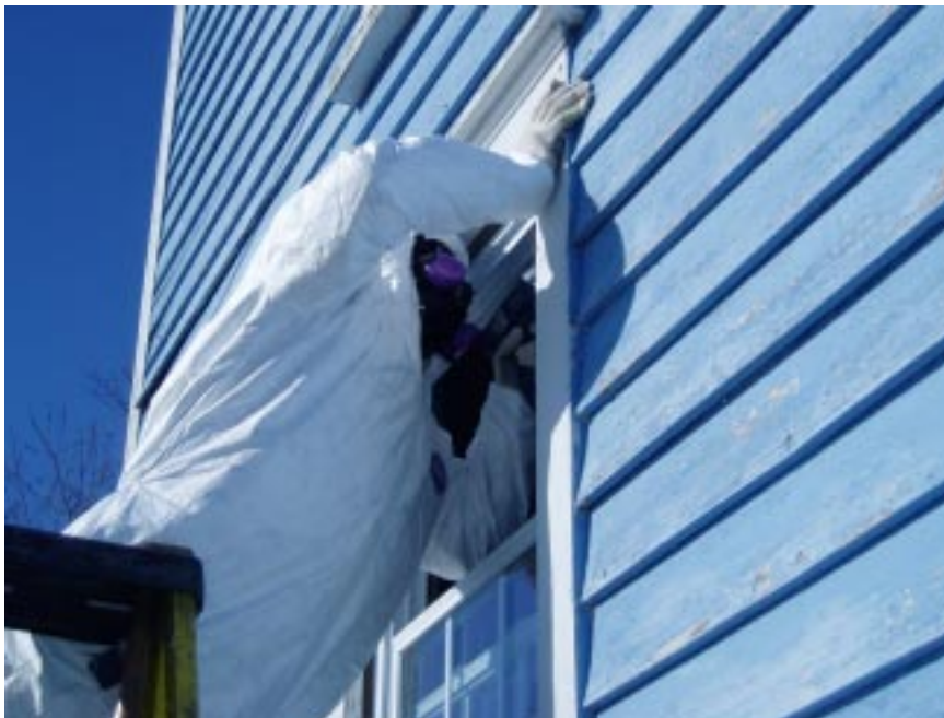
Certified Lead Contractor Worker Using Lead Safe Work Practices
