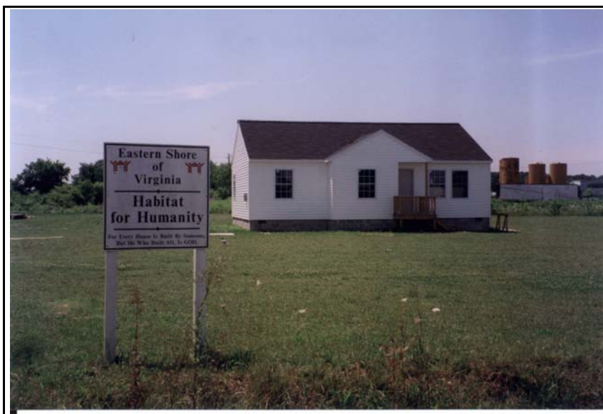
Habitat Home at Sunnyside Village
