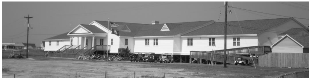
FIGURE 14.5 The Tangier Combined School was elevated in 2006 to mitigate flooding damages. Photo by Curt Smith
