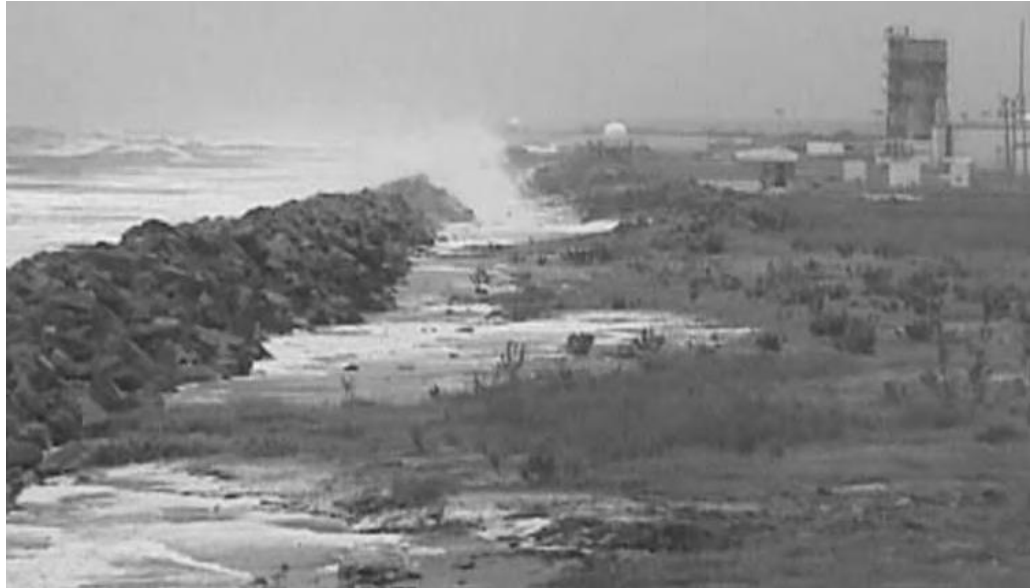
FIGURE 8.3 Waves overtopping the seawall on Wallops Island during Hurricane Dennis in September 1999. Photo Courtesy of U.S. Army Corps of Engineers.
