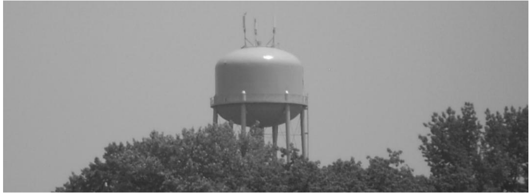
FIGURE 20.4 The Exmore Water Supply Tower supplies potable water to the Town's residents and businesses. Photo by Curt Smith.
