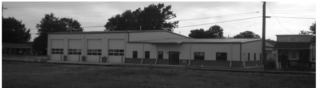
FIGURE 12.4 The new Fire and Rescue Department under construction in 2011. The railroad is a vital and historic component of the Town and can be seen in the foreground. Photo by Curt Smith
