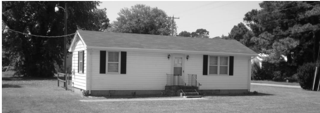
FIGURE 18.2 The Keller Town Office is at risk from storm water flooding and wind damage. Photo by Curt Smith
