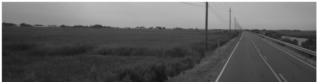
FIGURE 10.2 View of the causeway leading westward to Saxis. The causeway is the sole access to the island and is commonly flooded during storm events putting residents at risk. Photo by Curt Smith
