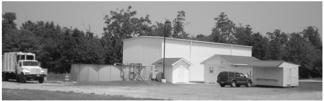
FIGURE 20.5 Exmore has two public sewer systems. The one shown was recently constructed in 2006 to serve Town residents and businesses. Photo by Curt Smith.
