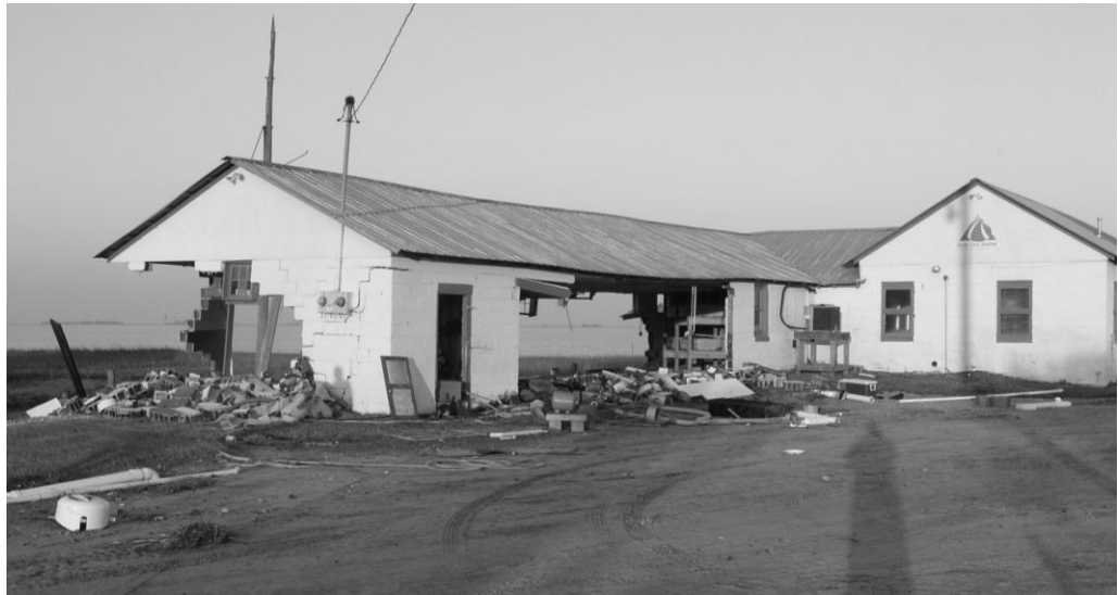
FIGURE 19.2 The Ocean Cove Seafood building in Magotha was destroyed during Hurricane Isabel in 2003. The 80 year old building had survived numerous storm events including the great hurricane of August 1933. At the time of its destruction, this seafood facility employed five people. Photo courtesy of Northampton County.
