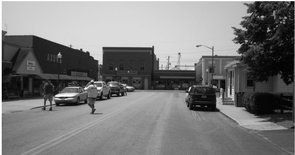
FIGURE 13.1 The Downtown Business District in Parksley is regularly flooded during larger rain events because the drainage pipes in this area are undersized. Rainwater commonly becomes backed-up as result and floods the streets and storefronts. Photo by Curt Smith.
