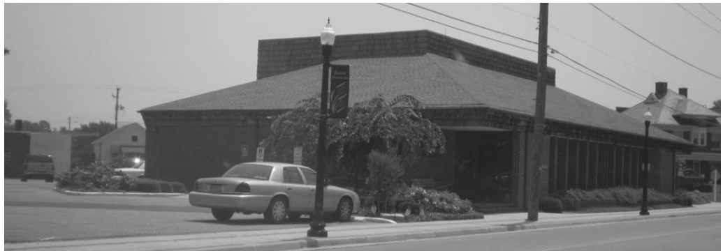
FIGURE 20.3 The Exmore Municipal Building is home to the Town Office and Police Department. Photo by Curt Smith.
