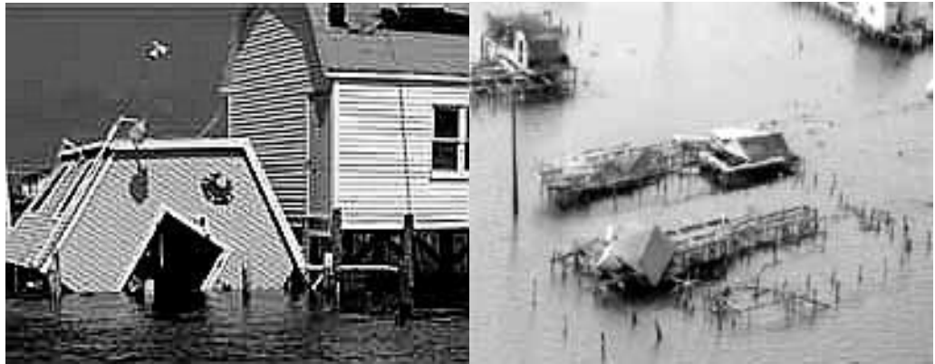
FIGURE 14.1 Crab houses on Tangier damaged during Hurricane Isabel. Left Photo by George Roarty, Right Photo by Chesapeake Fire Department
