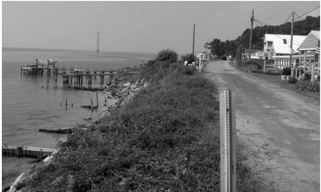
FIGURE 19.5 View of the eroded bluff and hardened shoreline protecting the small-cottage community of Silver Beach. Photo by Peter Stith.
