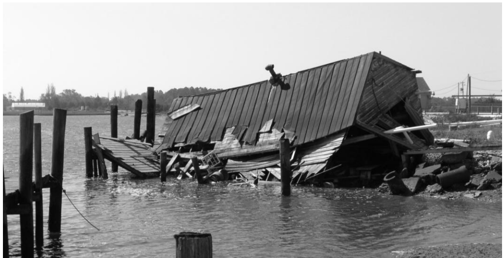
FIGURE 19.3 Older facilities are common along shorelines in the County and are more vulnerable to damage from coastal flooding. Photo courtesy of Northampton County.
