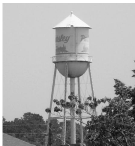
FIGURE 13.2 The Parksley Water Tower is the water source for Town residents. Wind is the greatest hazard threatening the structure. Photo by Curt Smith.
