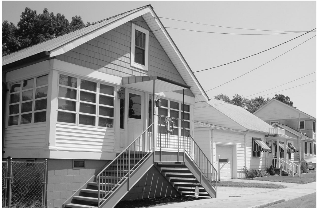
FIGURE 9.2 Chincoteague home elevation project.
