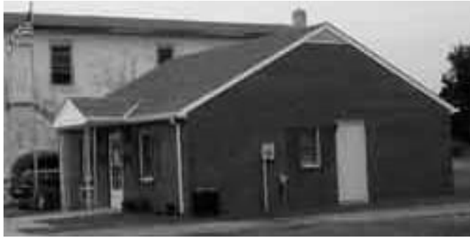
FIGURE 16.1 Photograph of the building that houses the Onley Town Office and Police Department. Photo by Ann Devletian, 2003-04.
