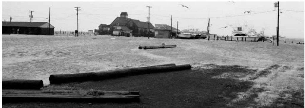
FIGURE 15.2 Photograph showing the surge from Hurricane Isabel in September 2003 impacting the same area depicted in Figure 15.1. Photo by Dan Bilicki
