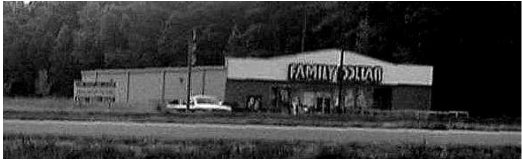
FIGURE 8.1 This building and its parking lot in Tasley frequently are flooded by storm water. As can be seen from the truck in the picture this building was built in a substantial depression. Just visible in the photo is the platform for customers to access the store after a rain. Photo by Elaine Meil
