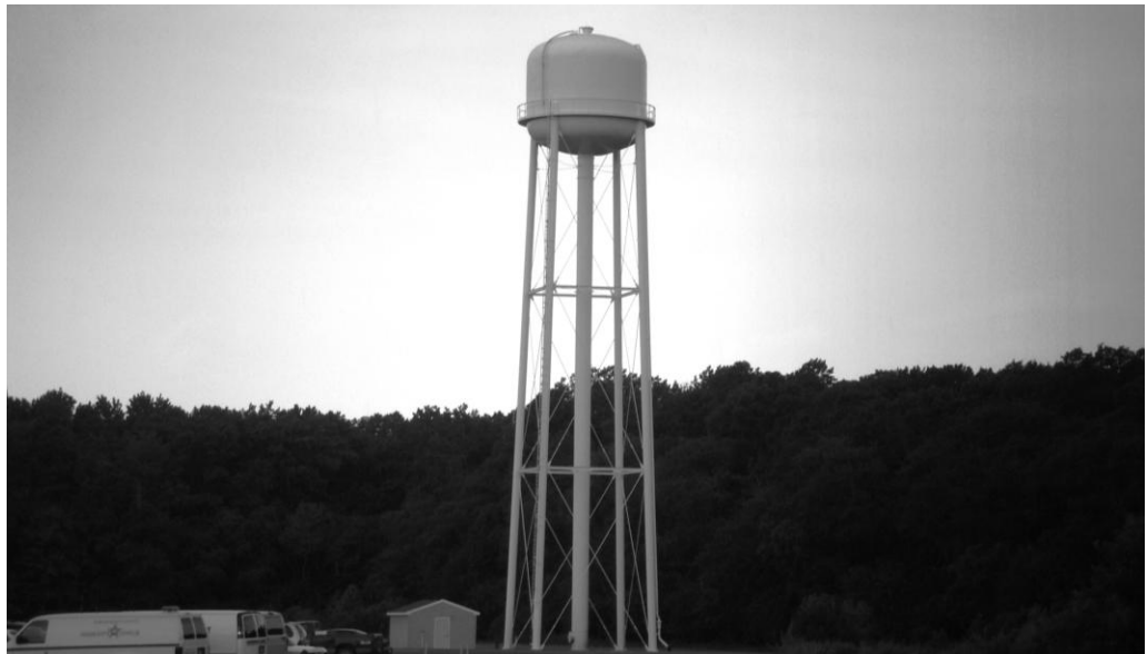
FIGURE 19.8 The Northampton County water tower in Eastville serves the County Courthouse Complex and is vulnerable to wind and ice damage Photo by Curt Smith
