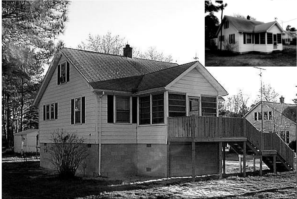
FIGURE 8.2 The County elevated this home in the Deep Creek area using Hazard Mitigation Grant Program money following Hurricane Floyd in 1999. Photos by David Fluhart
