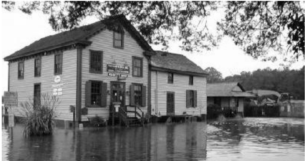
FIGURE 17.2 Photograph showing the historic Hopkins Store at the Onancock Wharf flooded during the November Northeaster of 2009. Commercial businesses are located in the two structures seen in this photo. Photo by Possum Lane
