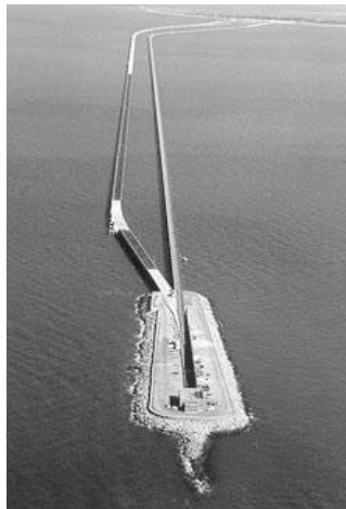
FIGURE 19.6 Chesapeake Bay Bridge Tunnel, the only southern road link to the Eastern Shore. Photo by Chesapeake Bay Bridge Tunnel Commission
