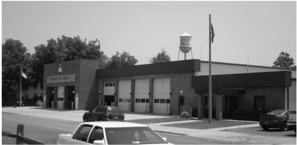
FIGURE 13.3 The Parksley Fire and Rescue Department services 7,500 people within Parksley and surrounding areas. Photo by Curt Smith.
