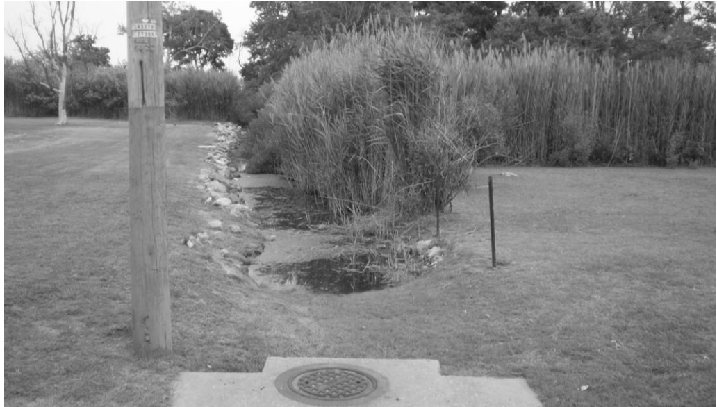
FIGURE 10.4 Drainage ditches in Saxis are commonly clogged by the invasive plant species, phragmites. Photo by Curt Smith
