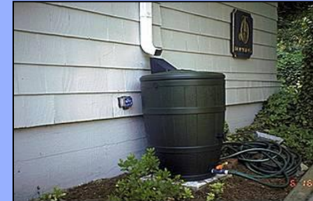
A rain barrel is used to collect rooftop runoff using a gutter/downspout system
