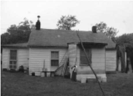
Substandard Home in Cats Bridge
