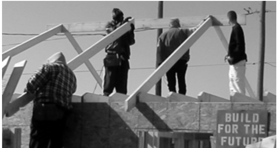
Build for the Future Trainees at work
