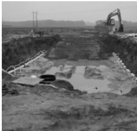
Bayview Sewer Construction
