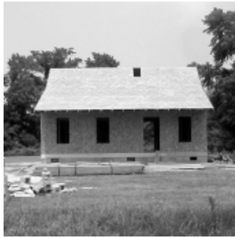
New Construction in Sunnyside Village
